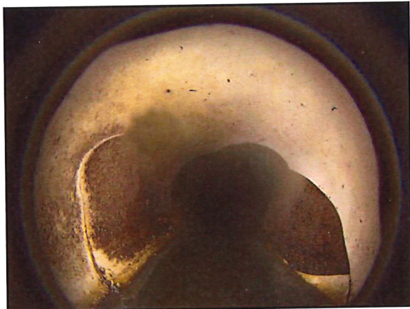
Figure 1: PS5_P077A; Condition: 5; Hole: Spot Repair
