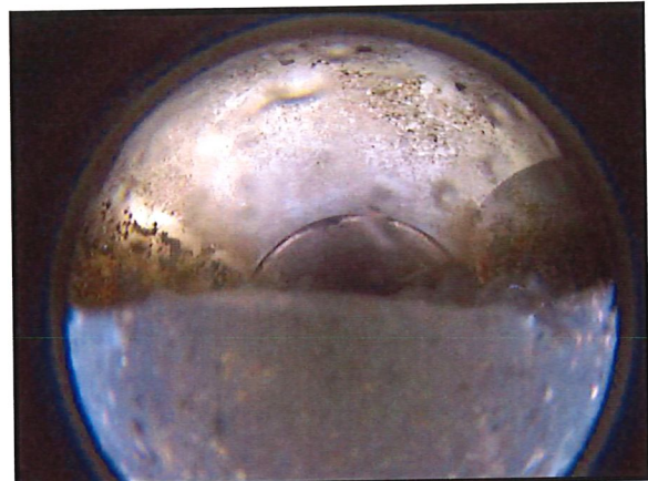
Figure 4: PS8_P048; Condition: 4; Water Level
