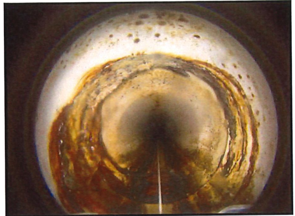
Figure 20: PS10_082A; Condition: 3; Encrustation
